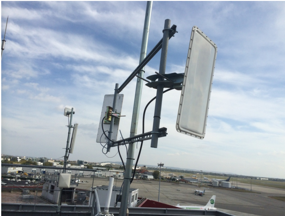
Figure 66: BS antennas implementation at the same height
