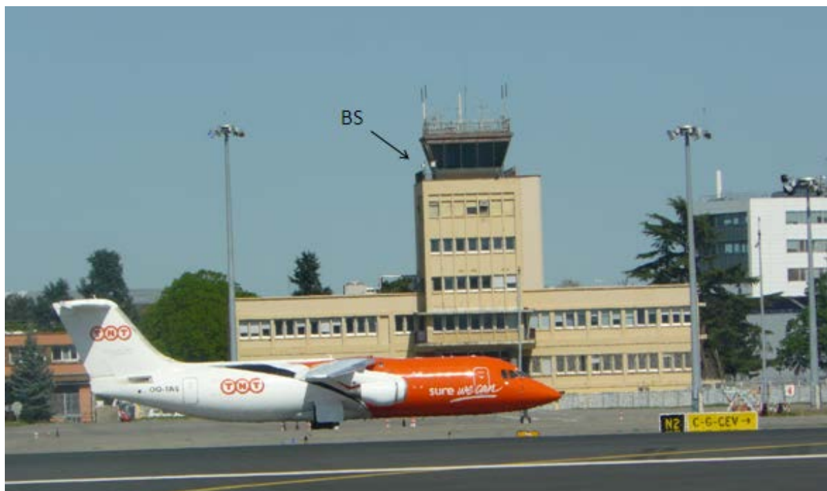
Figure 7-29: The former control tower with the 2 Thales BS
