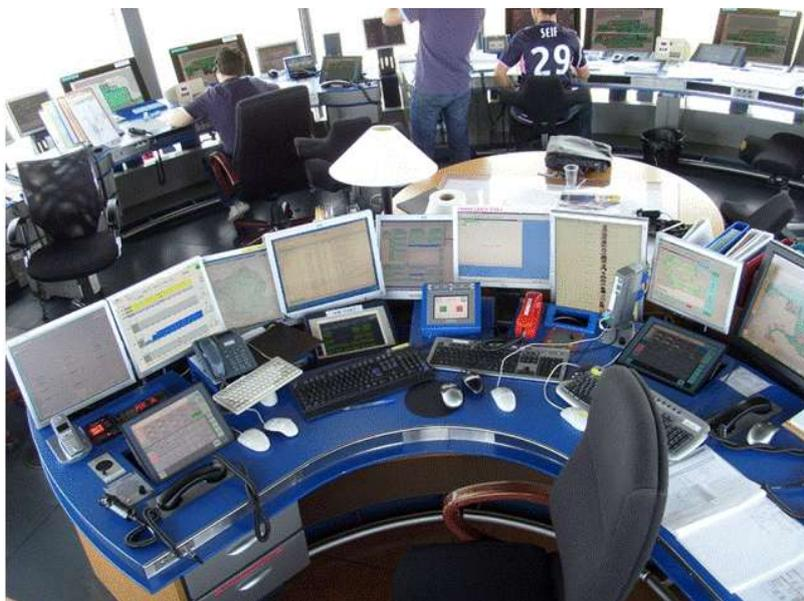
222 Figure 21: CDG - Tower Supervisor working position with the DMAN HMI on the left
