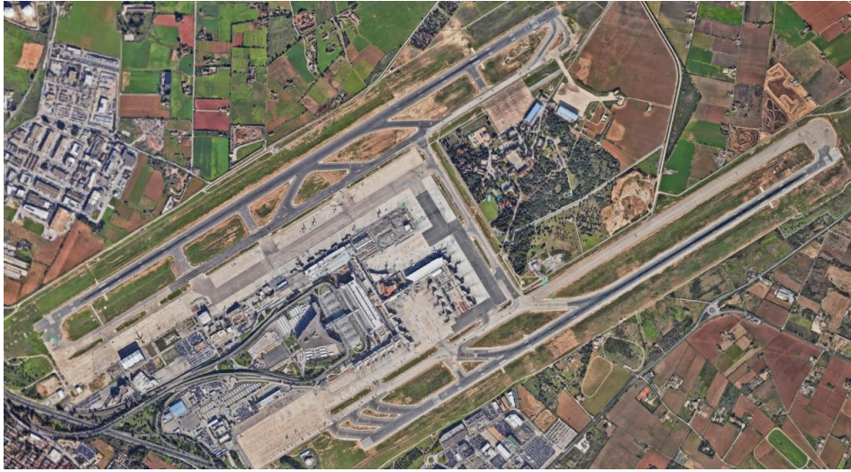
Figure 4. Plan view of Palma de Mallorca airport. Runway 06R is located at the South of the runway
